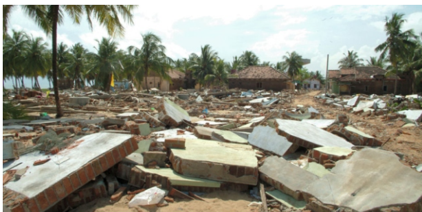
Devastation by the tsunami
